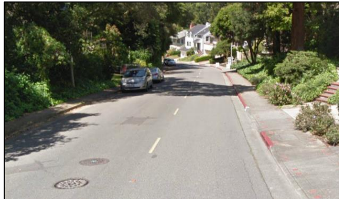
Figure 4. Trestle Glen Road - Westbound from Park Avenue
